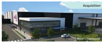
917 Boundary Road, Tarnet, VIC Completion 1H 2022 | Purchase Price $137.1m 1 GPT QuadReal Logistics Trust
