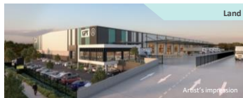
149 & 153 Coulson Street, Wacol, QLD GPT QuadReal Logistics Trust | Estimated End Value $40m 1
