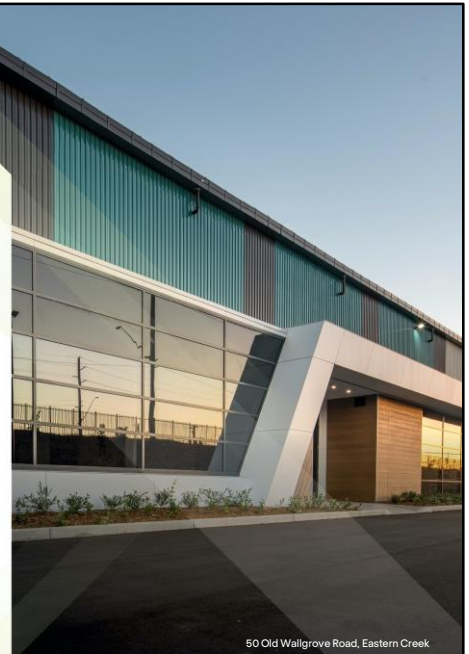
50 Old Wallgrove Road, Eastern Creek
