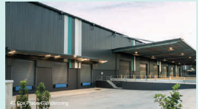
50 Old Wallgrove Road, Eastern Creek
