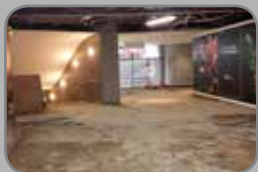
Retail redevelopment works commenced at the MLC Centre
